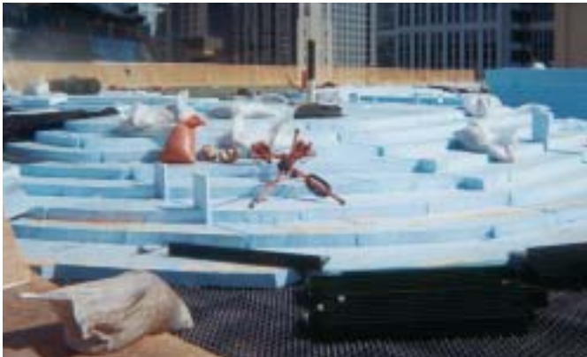
The roof garden, being installed above , incorporates a range of profiles ( top and below ) that differ in depth and type of growing media to accommodate existing features.
