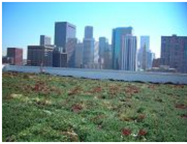
EPA building in Denver. Photo courtesy of GreenGrid Green Roof Systems.
