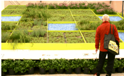
Chicago's Hyde Park Art Center has a greenroof of DIY modules, filled with growth and plant media, atop the Hyde Park Art Center building's existing roof. Photo by Robert Kravitz
