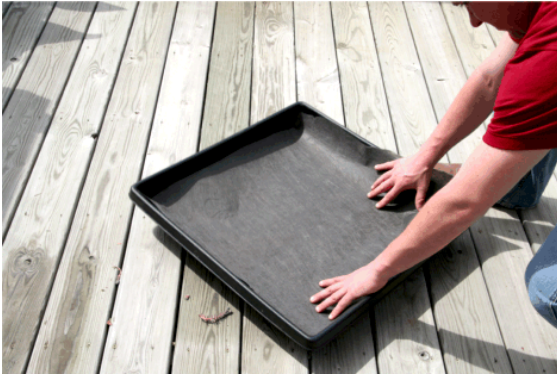
A soil filter fabric and root barrier is a necessary component to keep the drainage holes from clogging and to ensure non-penetration of any unwanted volunteer seedling taproots into the roofing membrane.
