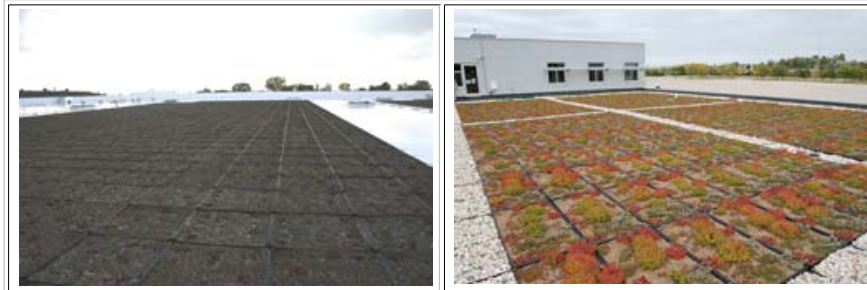
Photos, left to right: A Green roof modular system, recently planted. A Green roof and gravel system combined.
