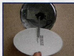
2 Attach cover plate to tension spring
