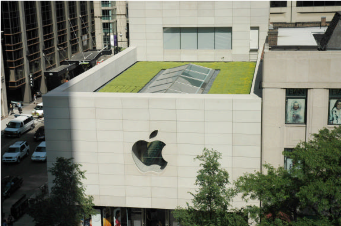
The Green Roof atop the Apple Store on Michigan Avenue, in Chicago, IL. See the case study in The Greenroof Projects Database here on Greenroofs.com here .
